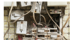
Switches and relays
